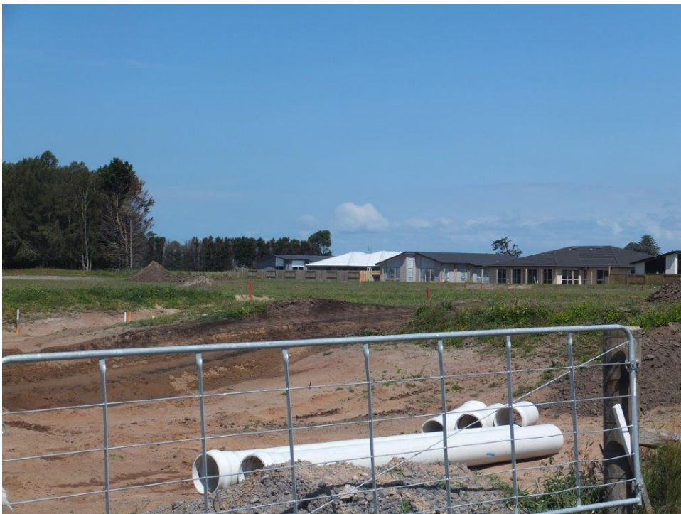
Figure 2 A greenfields SHA, showing earthworks and new homes.
